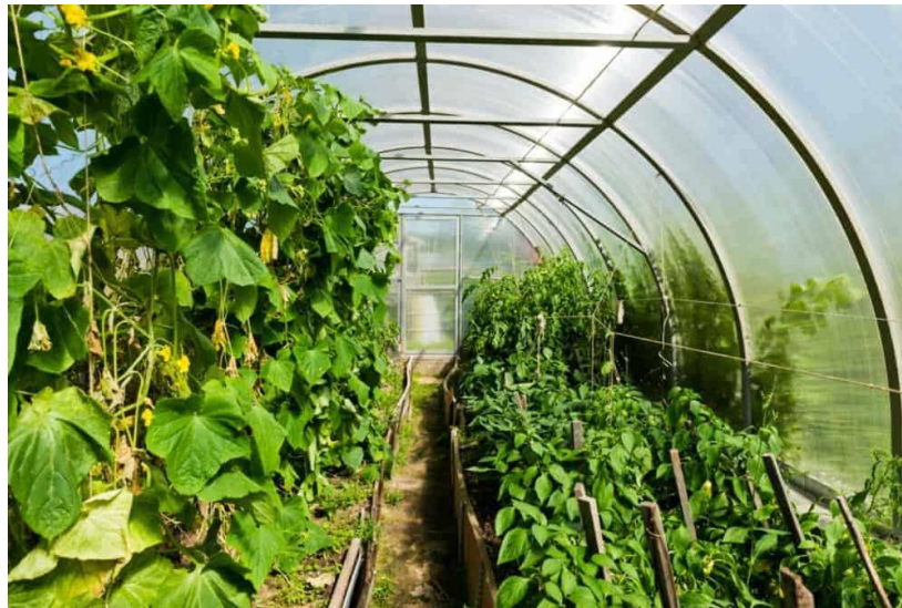
Figure 1. Rebuilt Greenhouse Structure in Mandalamekar Village
